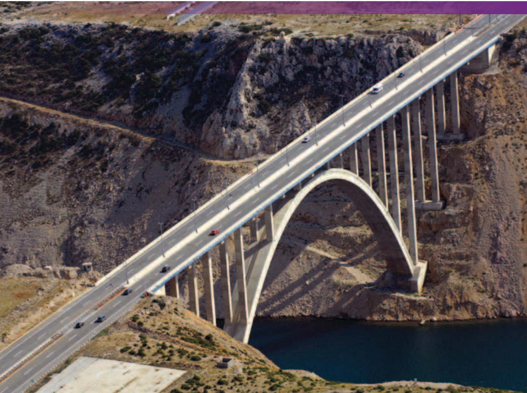
New Maslenica bridge (motorway A1)
