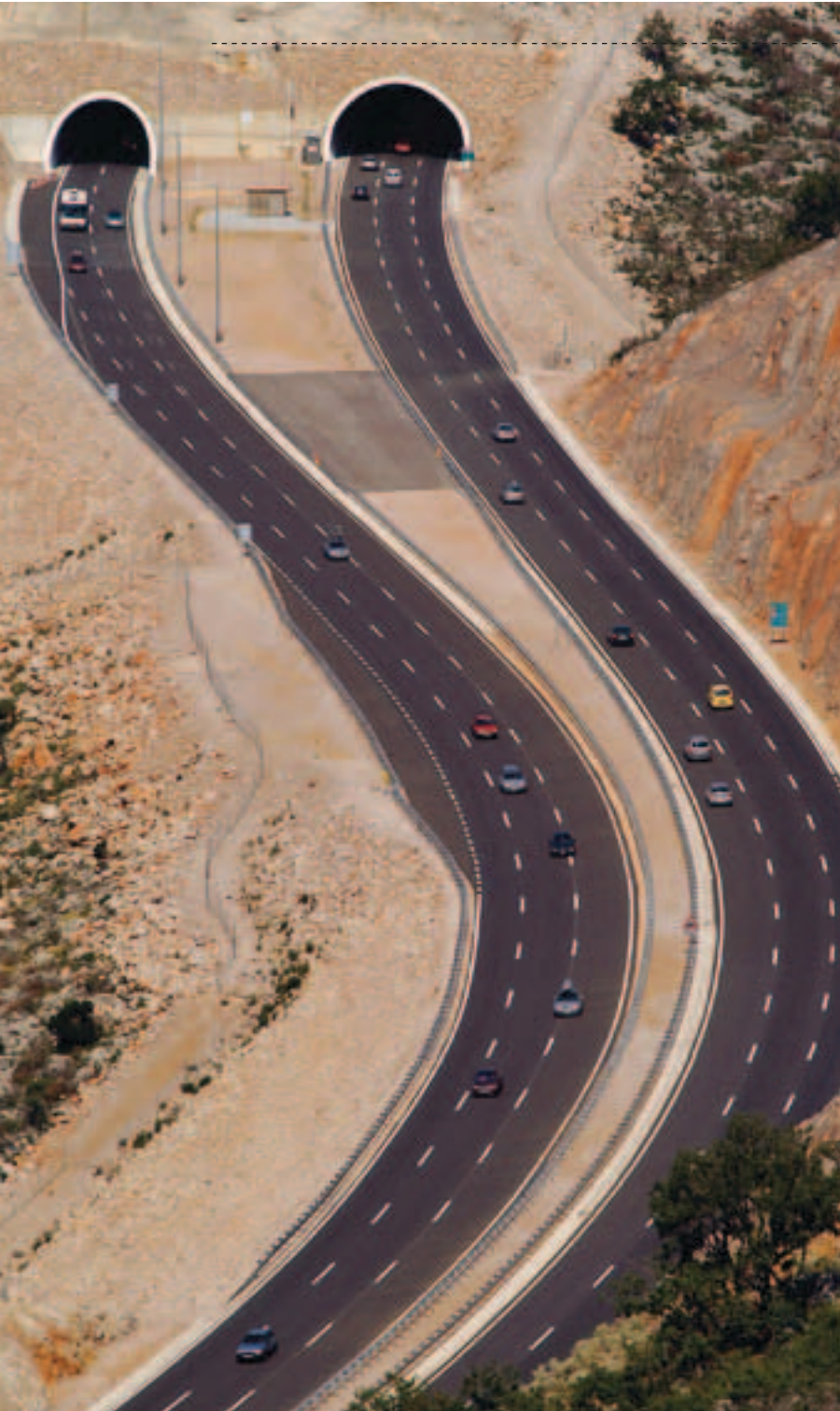
Tunnel Mala Kapela
